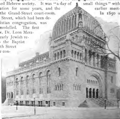
TEMPLE BETH-EL, HEBREW, FIFTH AVENUE AND 78th STREET, OPPOSITE CENTRAL PARK.
